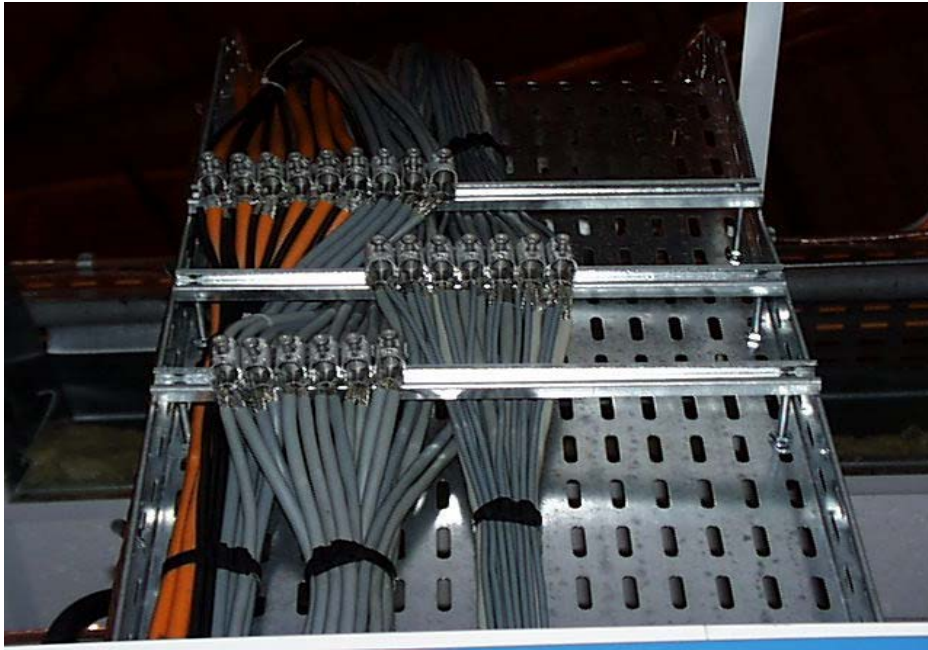
Figure 9.4 Spring clips installed on cables
